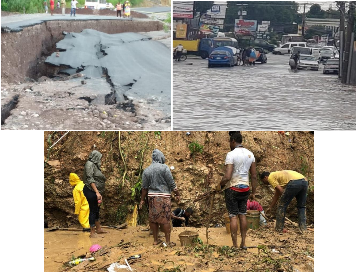
Figure 2-1: Disasters from 2020 rainfall Incidents (Damage in Junction roadway (top left); Kingston Roadway into rivers (top right); Death from landslides in Shooters Hill (bottom) (Source of Photos: Loop Jamaica)
