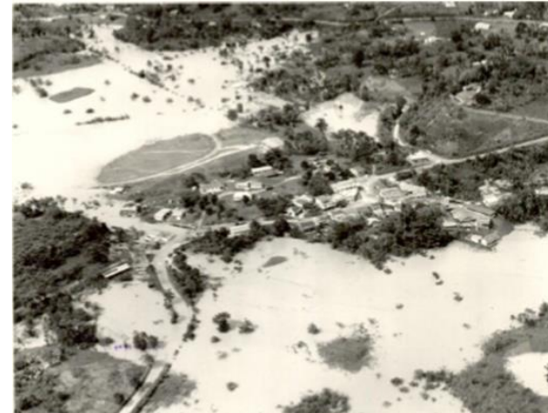
Flooding due to Hurricane Kate 1985 Source: New Market Agriculture Disaster Risk Management Plan, 2012
