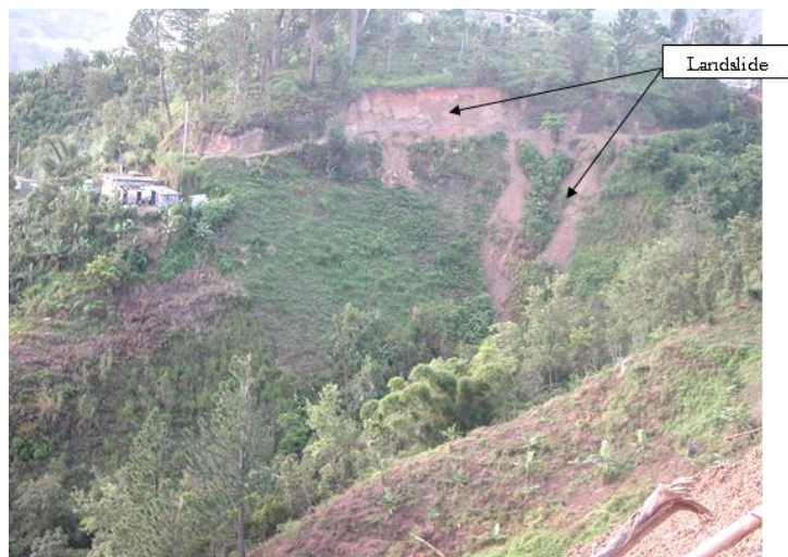
Photo 52: View of landslide in Penlyne Castle (Y-S road). Material has been dumped on the roadway to improve access. [Photo: M. Downswell]
