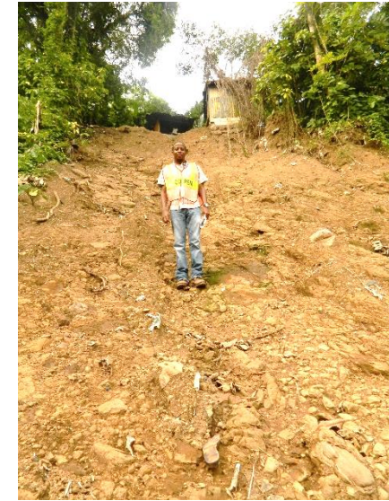
Landslide in Breastworks. Source: ODPEM.
