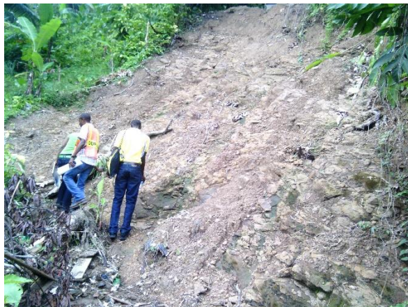
Landslide in Breastworks. Source: ODPEM.
