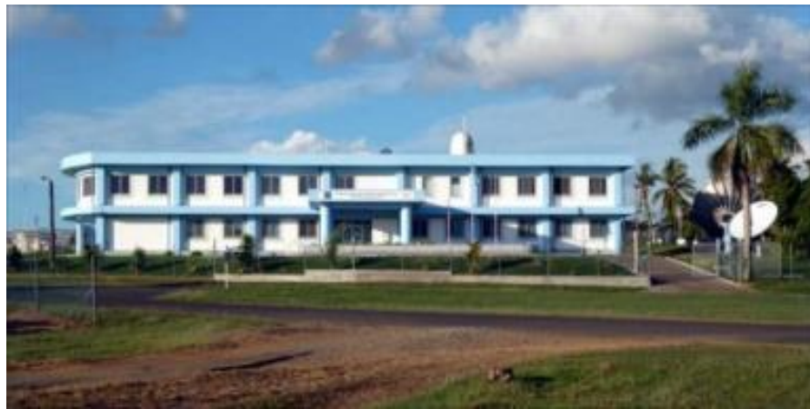
FMS Building in Nadi, May 2015 (The photo was taken by Mr. Koji Kuroiwa of JICA Expert)
