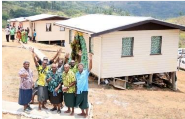
Tukuraki Village Relocation Project site, Ba
