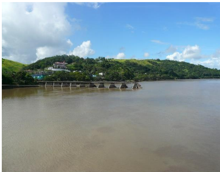
Sigatoka Bridge, January 2009
