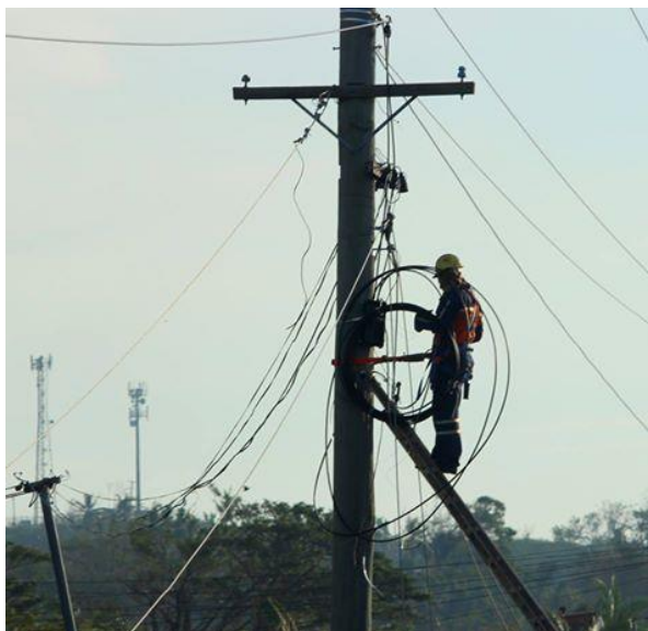
FEA Repairs, March 2016
