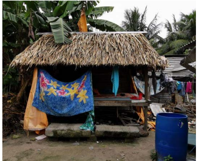
Cyclone and storm surge shelter - Kiribati Photo: Un Women/Rahel Steinbach
