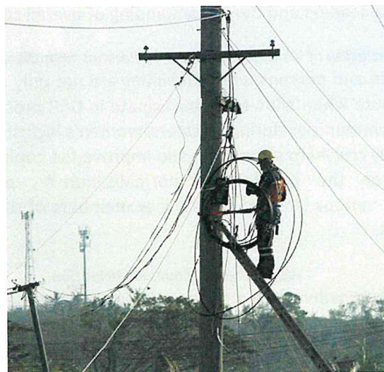
FEA Repairs, March 2016
