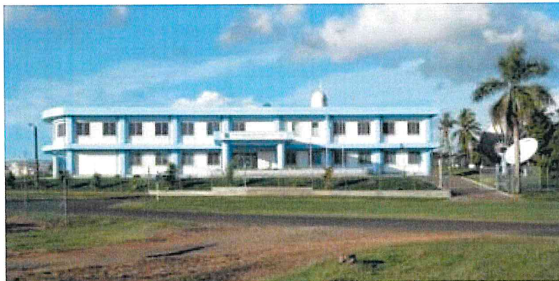
FMS Building in Nadi, May 2015 (The photo was taken by Mr. Koji Kuroiwa of JICA Expert)
