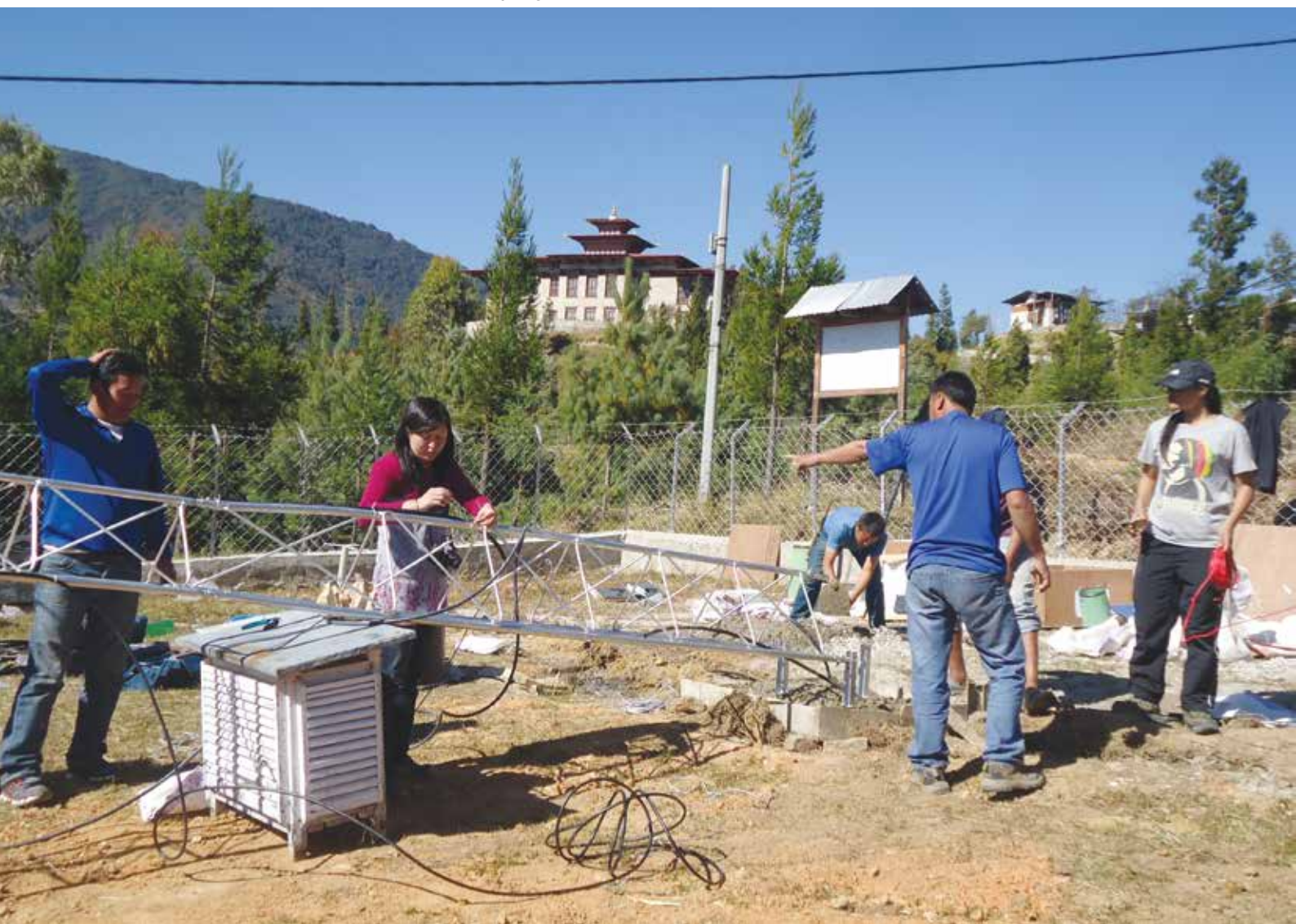
Automatic weather station installation at Trashiyangtse
