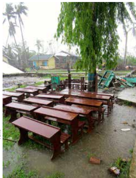
School damage in the Philippines.
