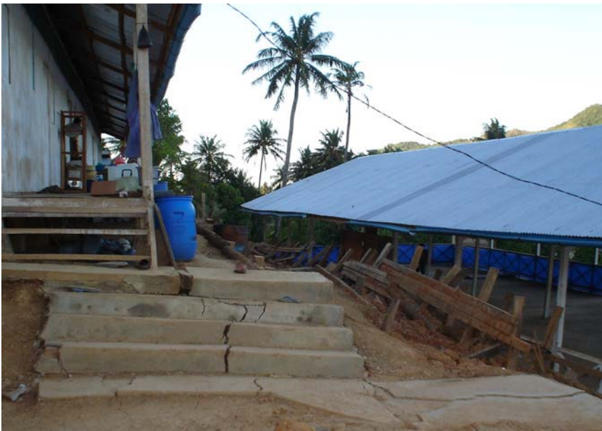
Temporary shelter built on hills damaged by landslides, Seibun Ketapang, Aceh
