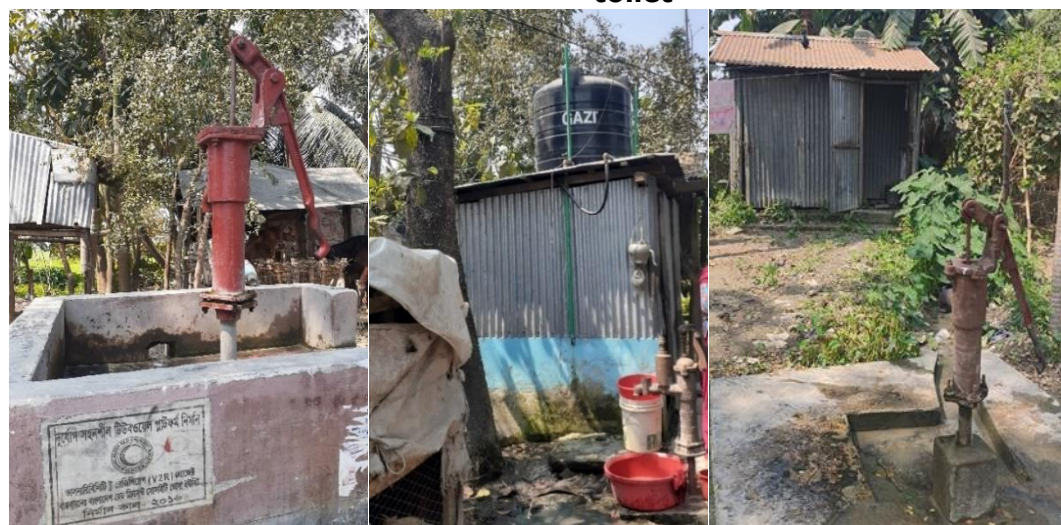
Picture 6: (a) Raised tube well (b) general tube well and bathroom (c) tube well and toilet
