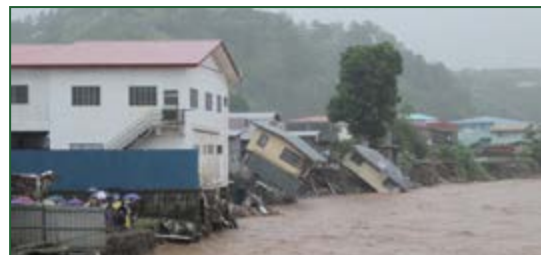
Figure 3: Severe flooding of the Mataniko River in April 2014
