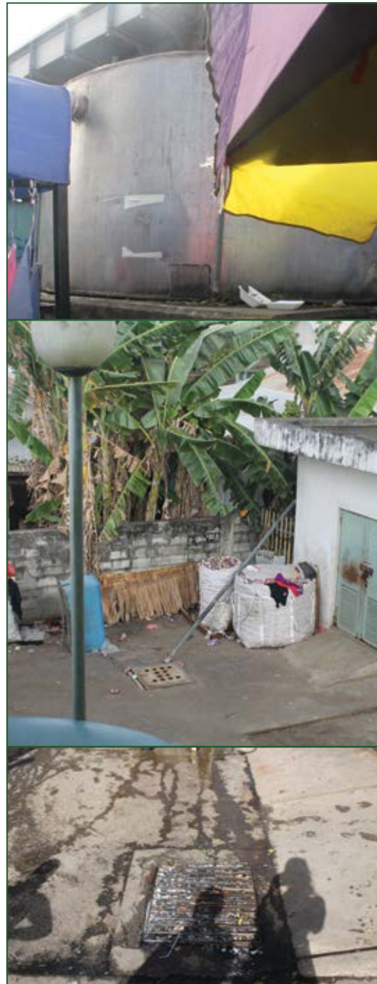
Figure 15, 16, 17: Disused rainwater tanks; disused electricity generator; blocked drainage system
