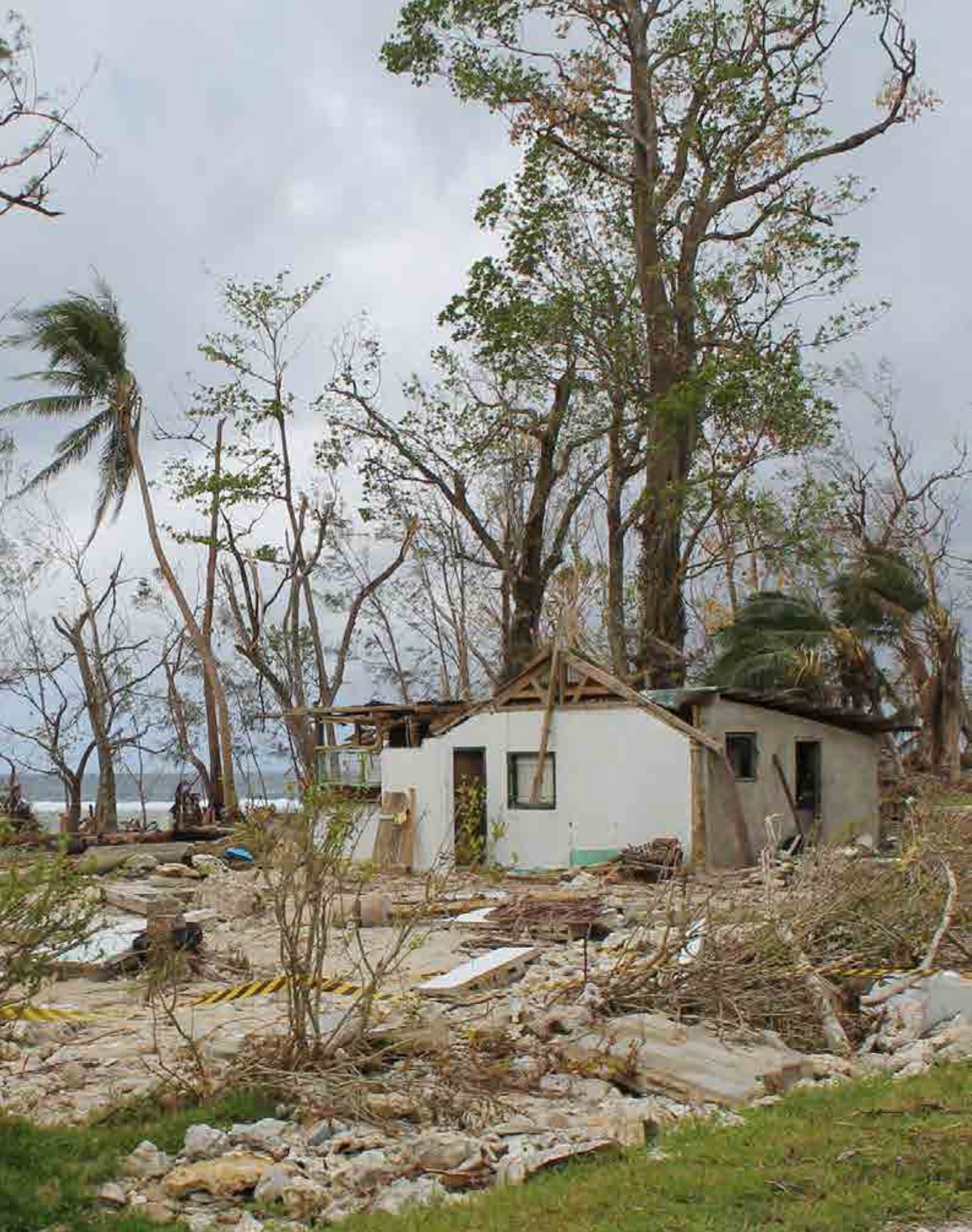
Efate Island (Vanuatu) -Some of the destruction caused by Cyclone Pam on the east coast of Efate Island in Vanuatu. Many people have not only lost their homes; they have also lost their crops - both their source of food and income.
