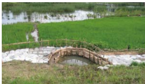
Fig.2 Dyke protected by a Yaing Khway
