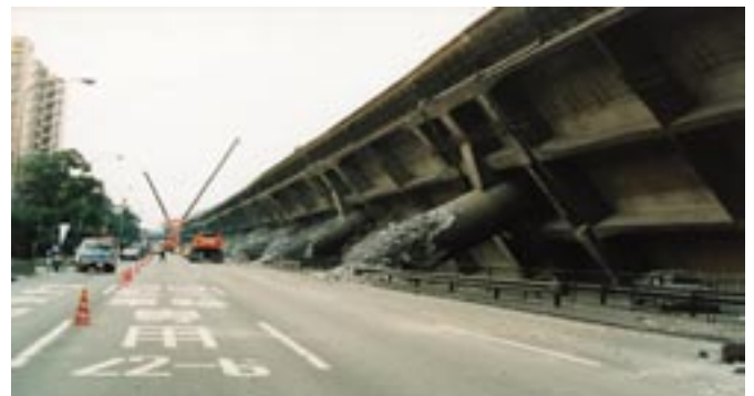
Restoring of the highway which collapsed in the Great Hanshin-Awaji earthquake: images before and after the reconstruction
