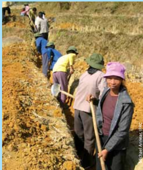
Constructing safe water supplies, Damian Village, Guangxi, China 2004.
