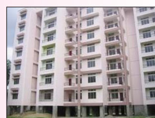
Fig. 3: Soft storey buildings as above are dotting everywhere as a mark of modern development. But their performance during Bhuj (2001) earthquake and many other countries, including Japan, Taiwan; signify that these are deficient structures. The importance of retrofitting them has appealed many to go ahead but experiences show that in the name of "jacketing" ground floor columns only, proper engineering is not ensured. It is rather better to go for selective "filling up" of open frame/bay at such floors by simple full width brick walls that may not obstruct parking or other functionalities.
