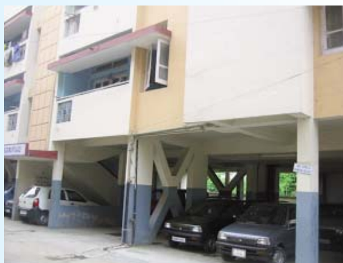
Fig. 3: Soft storey buildings as above are dotting everywhere as a mark of modern development. But their performance during Bhuj (2001) earthquake and many other countries, including Japan, Taiwan; signify that these are deficient structures. The importance of retrofitting them has appealed many to go ahead but experiences show that in the name of "jacketing" ground floor columns only, proper engineering is not ensured. It is rather better to go for selective "filling up" of open frame/bay at such floors by simple full width brick walls that may not obstruct parking or other functionalities.
