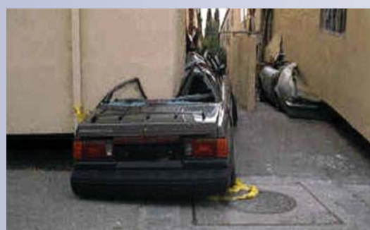
Fig. 2: If cars are found crashed in this manner under stilt floor for the very simple yet important lacuna in building construction, it's high time to adopt correction measures as per expert advice. The construction of buildings with "soft storey" for the urgently needed parking space at the ground floor can be facilitated following simple retrofitting as envisaged in this note.
