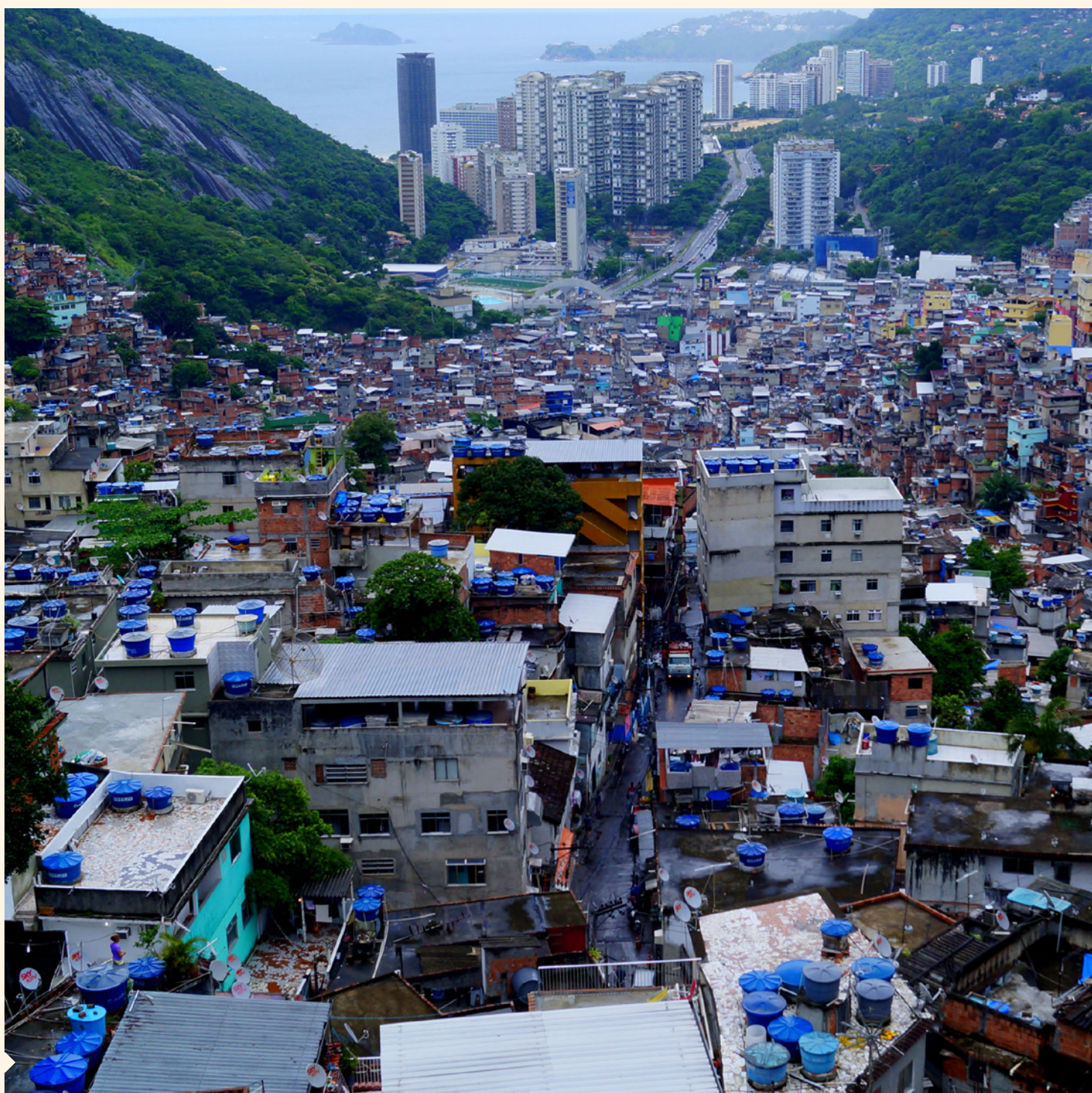
Aerial view of water tanks on the rooftops of Rocinha slum in Rio de Janeiro, Brazil
