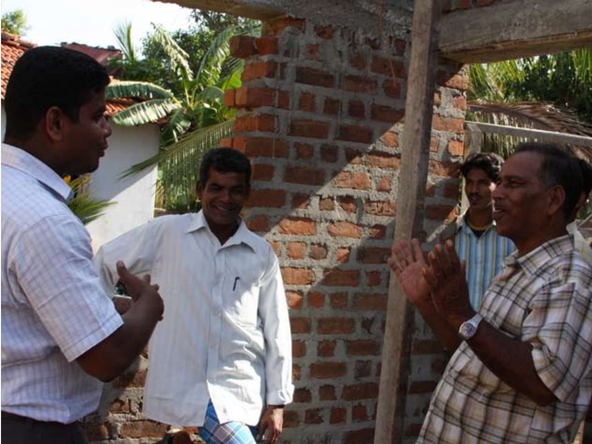
A Home owner, UN-HABITAT staffer and masons discuss the progress of construction
