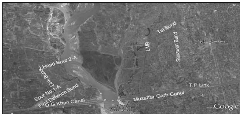
Figure 4: Taunsa Barrage – Flood Protection Infrastructure
