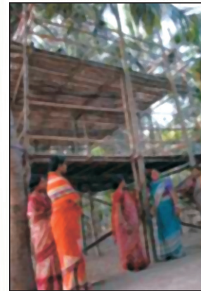
Fig. 24: Maachas built in West Bengal by local disaster preparedness committees to replicate traditional flood coping methods across the border in Bangladesh
