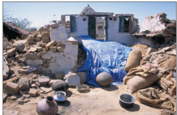
Fig. 3: Carpenter Nila Bhai Norgha's house, destroyed by the earthquake in Gujarat
